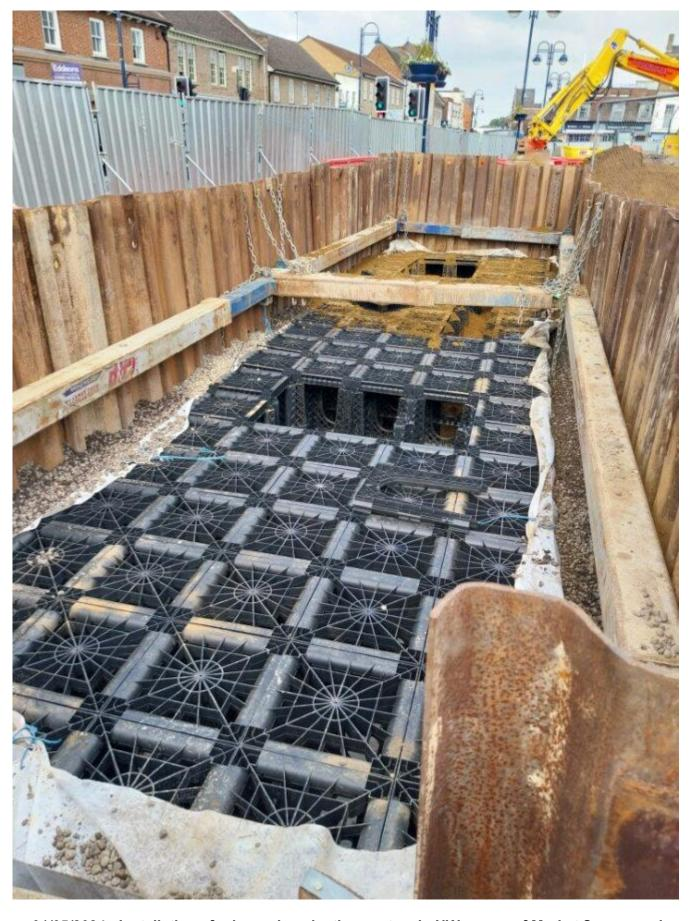
01/05/2024 - Installation of rain garden planting system in NW corner of Market Square and backfilling.
