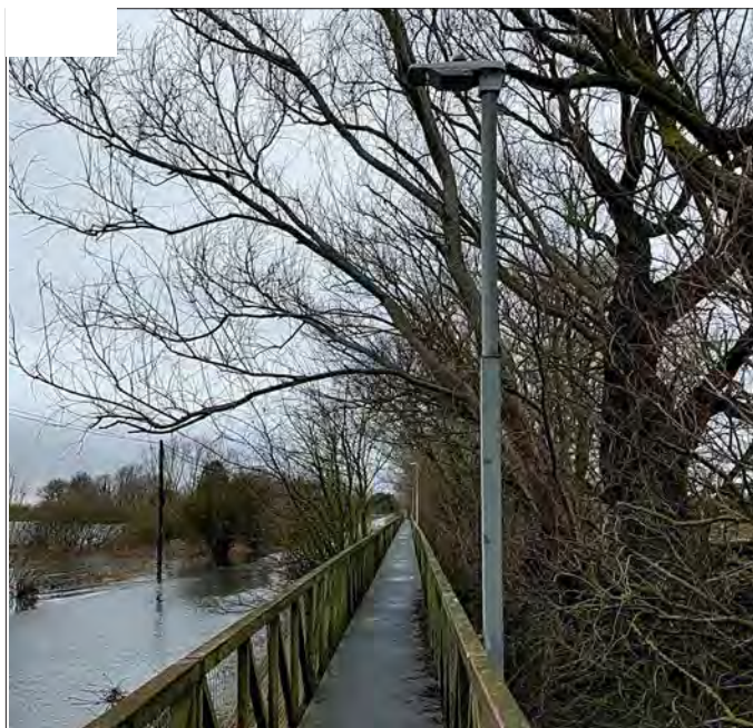
25c: Pedestrian raised walkway and lighting
