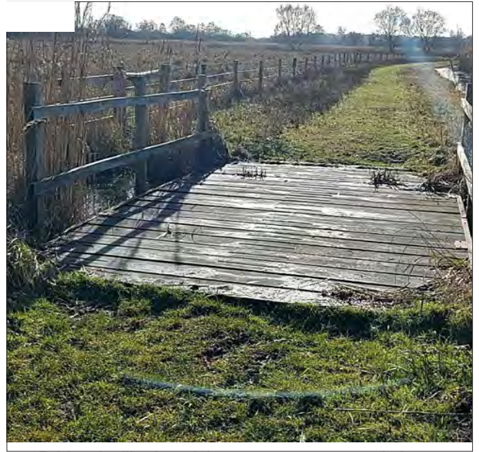
8a: Bridge facilitating visitor movement around site
