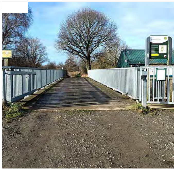
1b: Bridge onto the site and information signage
