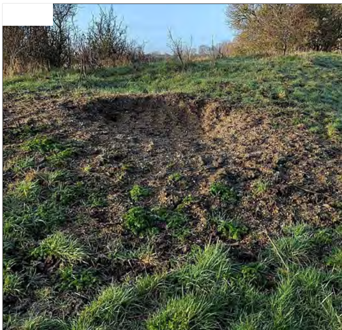
21: Erosion and exposure of bare ground
