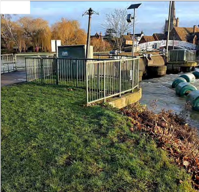
5: Bridge and sluice over Great River Ouse
